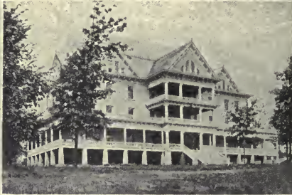
IOWA SANITARIUM, NEVADA, IOWA.
